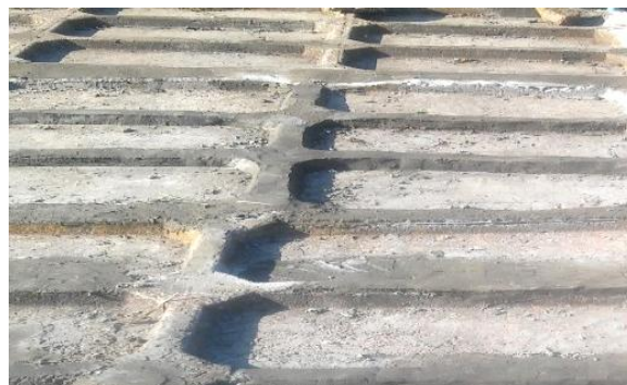
Fig. 5. The pre-chamber panels after structural repair
