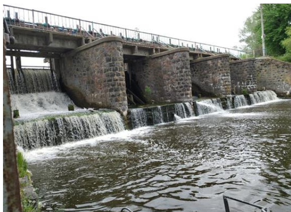
Figure 1. Hydraulic facility of the Fastiv Reservoir
