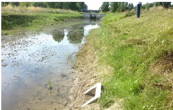
Fig. 10. Technical condition of the MK-28 open channel and restoration of the mouth of the closed collector at DK-1 on the Melnytska DS
