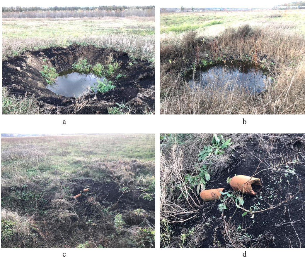
Fig. 5. Consequences of military actions in the area of the Irpinska DMS: a – a crater from a shell, shown on a satellite image (see Fig. 4 a); b – grass overgrowth of the craters over time; c – closed drainage network damaged by explosions; d – fragments of tile drainage (photos by A. Shevchenko)
